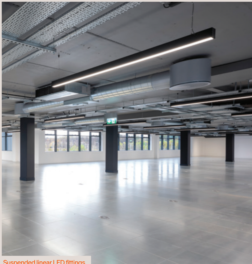
Suspended linear LED fittings
