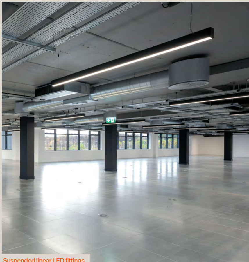
Suspended linear LED fittings
