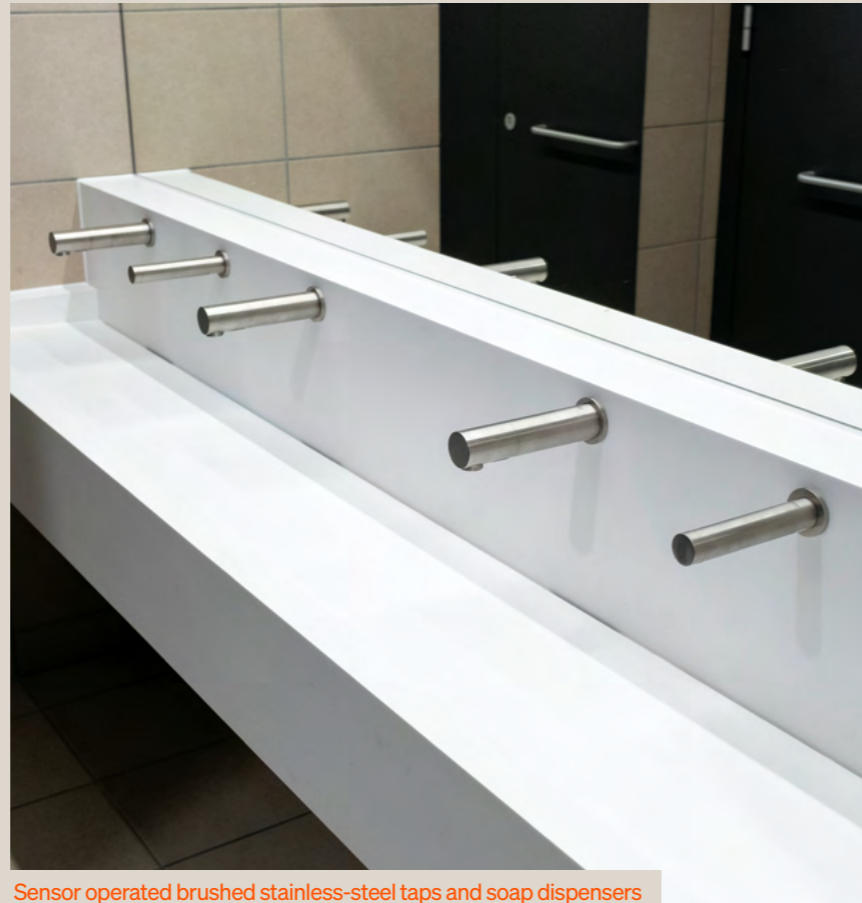
Sensor operated brushed stainless-steel taps and soap dispensers
