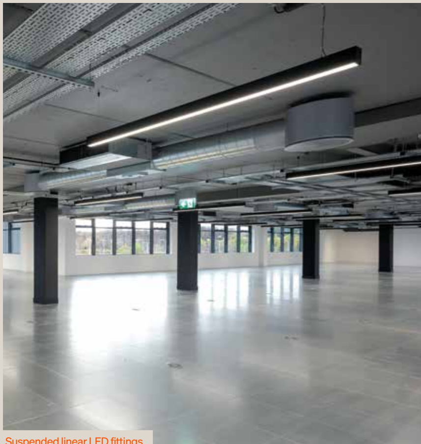
Suspended linear LED fittings
